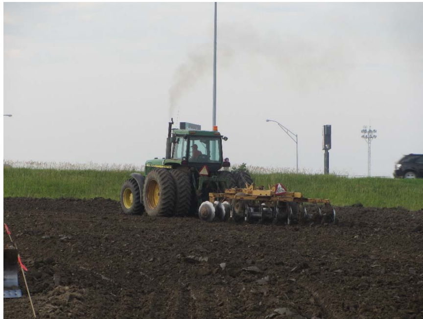
Figure 103. Pottawattamie County Project 6: Disc cultivator used to dry embankment materials
