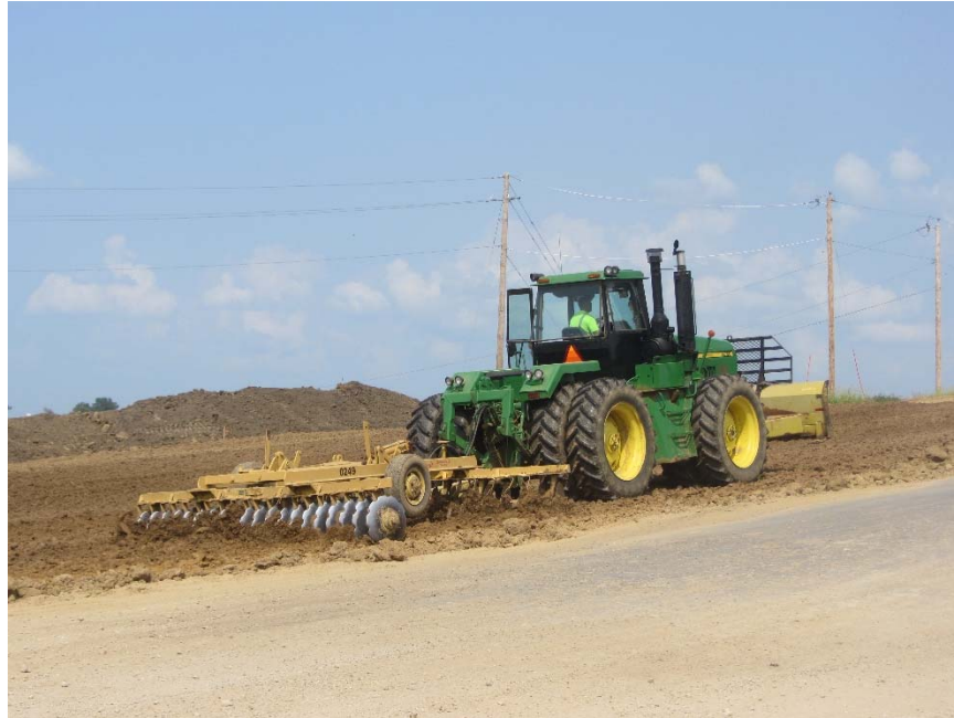
Figure 128. Scott County Project 8: Disc cultivator used to dry embankment materials
