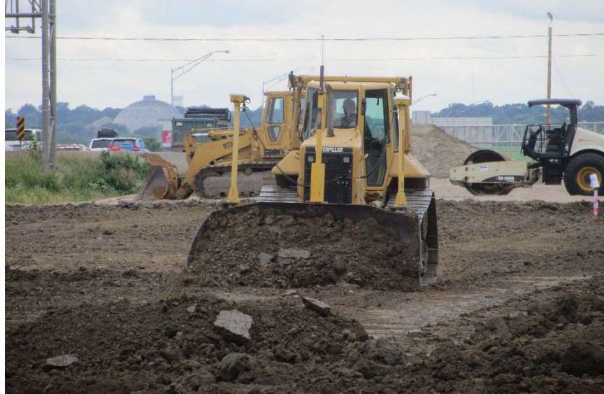
Figure 100. Pottawattamie County Project 6: Caterpillar dozer used to control lift thickness
