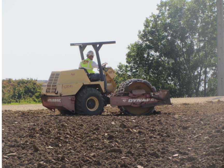
Figure 130. Scott County Project 8: Dynapac padfoot roller used for soil compaction
