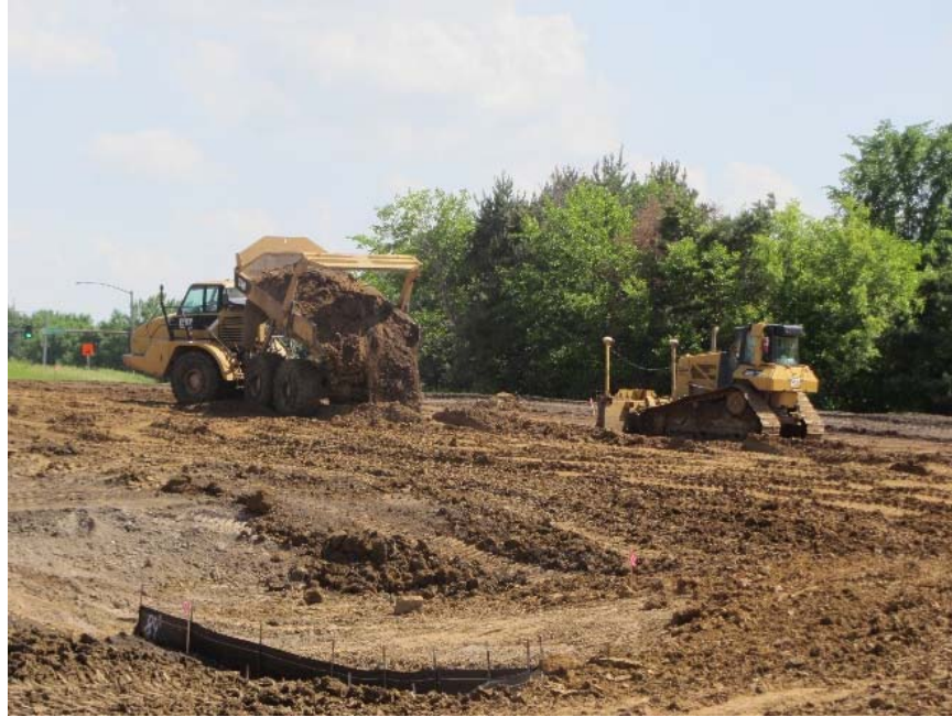
Figure 74. Lynn County Project 4: Caterpillar 740 dump truck used to place loose fill materials
