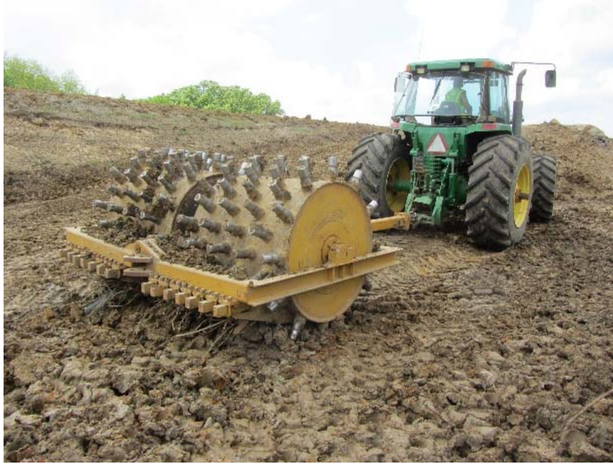
Figure 26. Polk County Project 1: Pull-behind sheepfoot roller used for soil compaction
