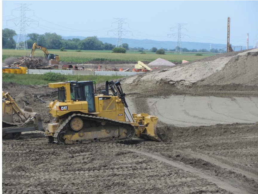
Figure 113. Woodbury County Project 7: Caterpillar D6T dozer used to control lift thickness
