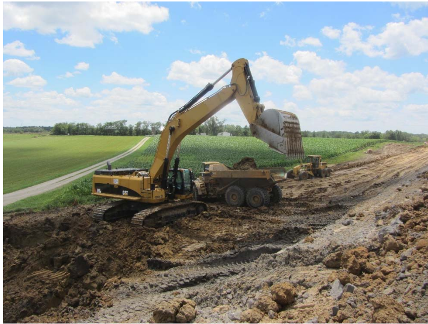
Figure 52. Linn County Project 3: Caterpillar 390D excavating material from borrow source
