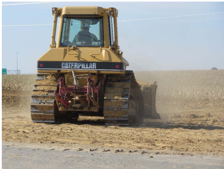
Figure 127. Scott County Project 8: Caterpillar dozer used to control lift thickness
