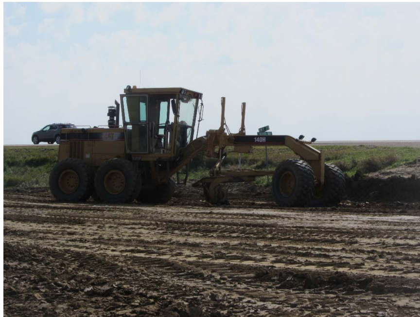
Figure 143. Woodbury County Project 9: Caterpillar 140H motor grader used to level the embankment surface
