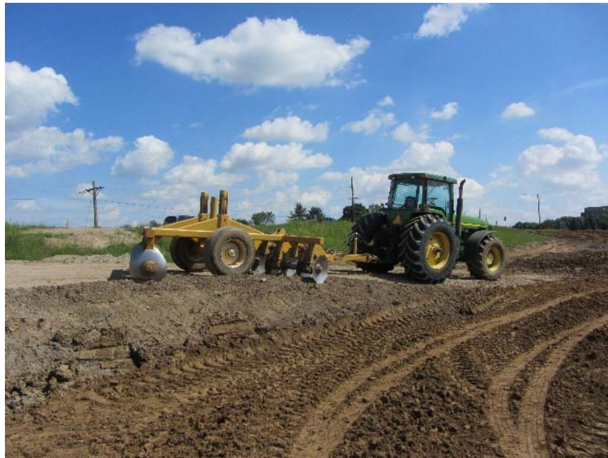
Figure 79. Linn County Project 4: Disc cultivator used to dry embankment materials
