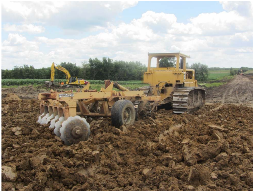
Figure 54. Linn County Project 3: Disc cultivator used to dry embankment materials
