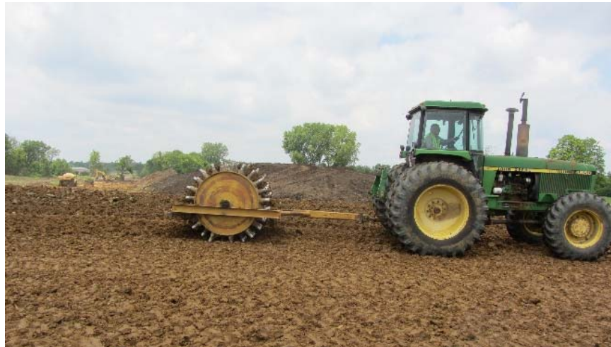
Figure 75. Linn County Project 4: Sheepfoot roller used for soil compaction
