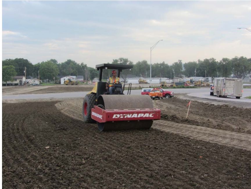
Figure 102. Pottawattamie County Project 6: Dynapac CA250-II vibratory smooth drum roller used for soil compaction
