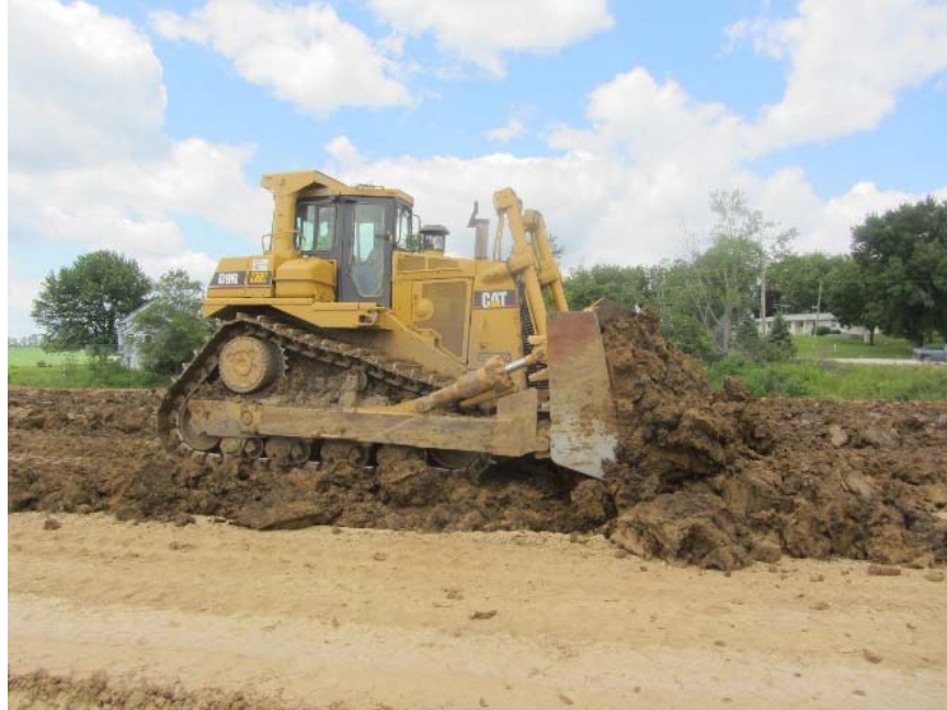
Figure 53. Linn County Project 3: Caterpillar D6R dozer used to control lift thickness
