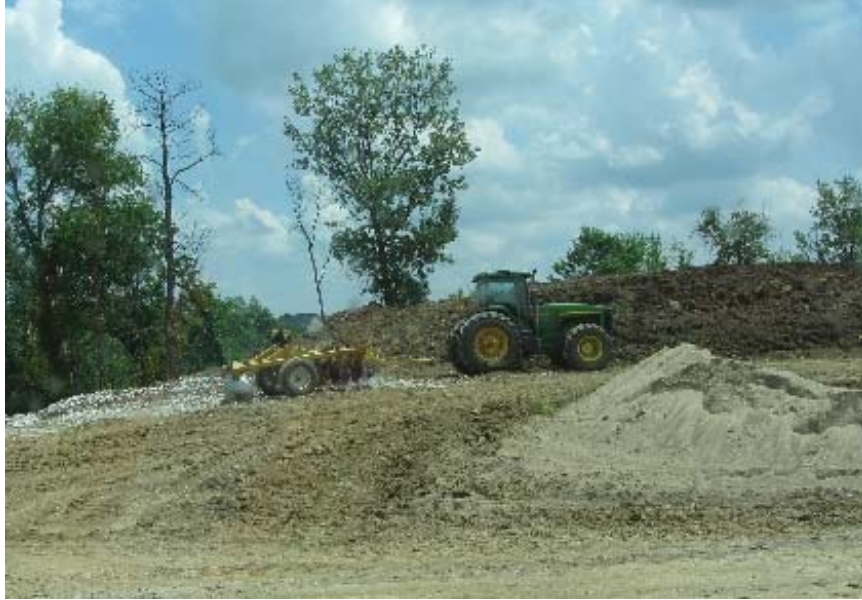
Figure 24. Polk County Project 1: Disc used to dry embankment materials
