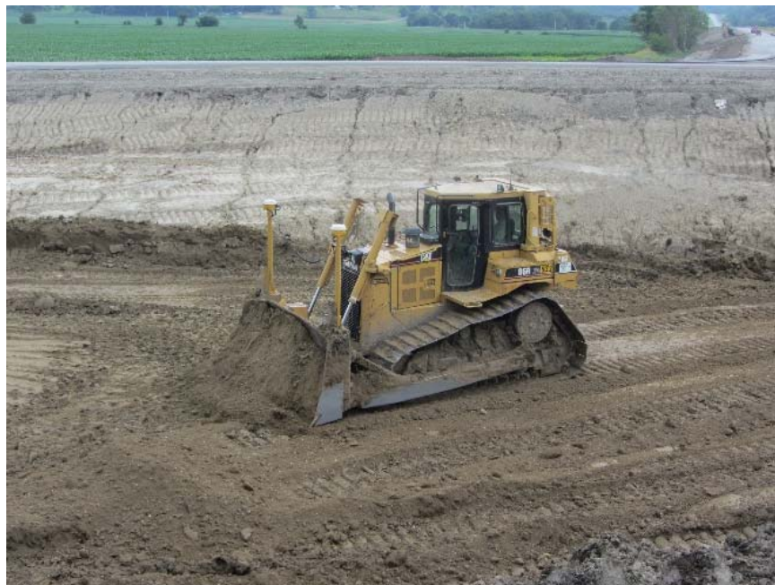
Figure 89. Mills County Project 5: Caterpillar D6R dozer used to control lift thickness
