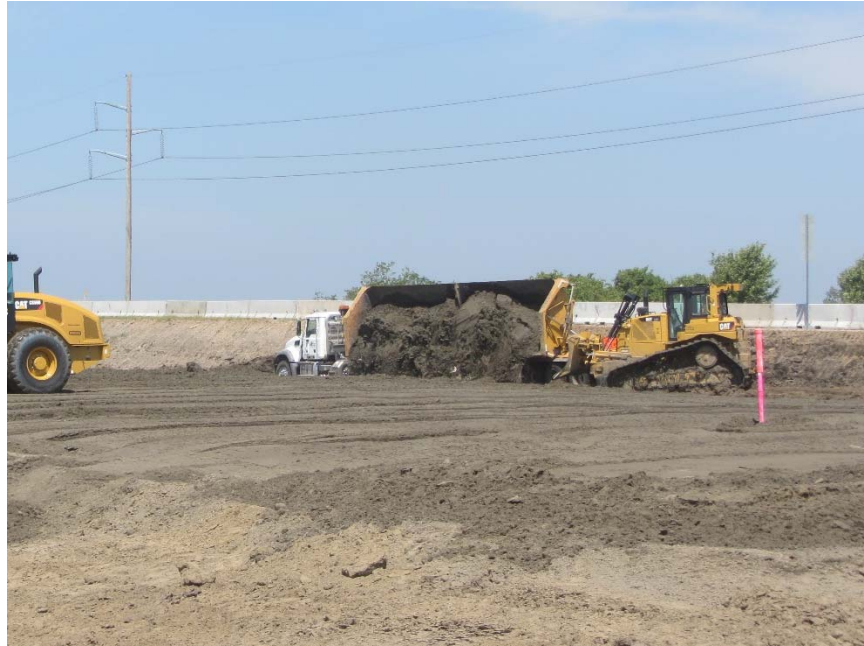
Figure 112. Woodbury County Project 7: Dump truck used to place loose fill materials
