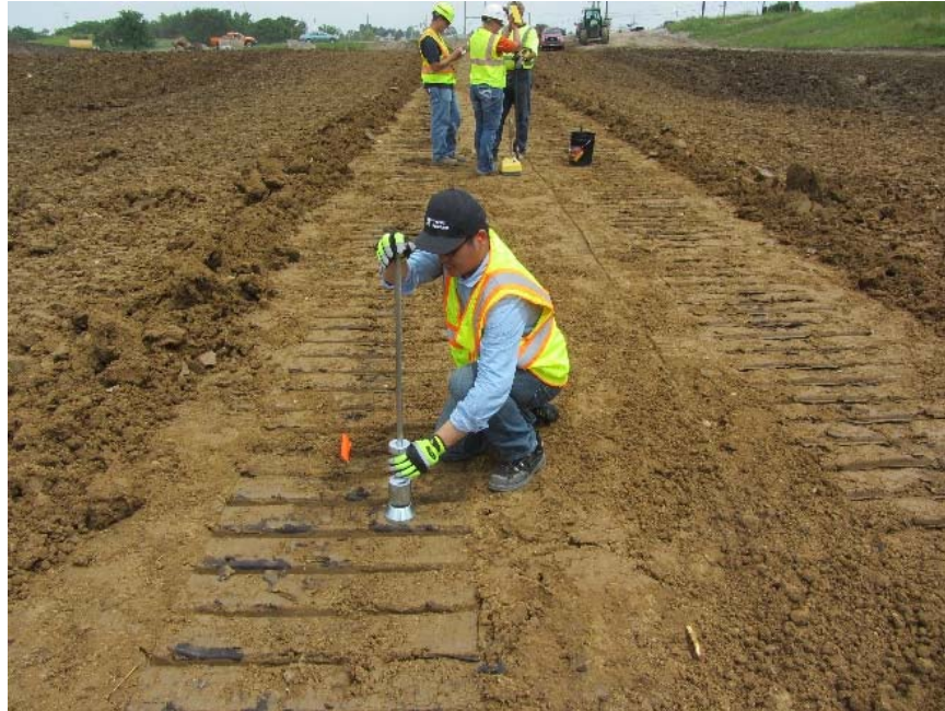
Figure 78. Linn County Project 4: ISU in situ drive cylinder test
