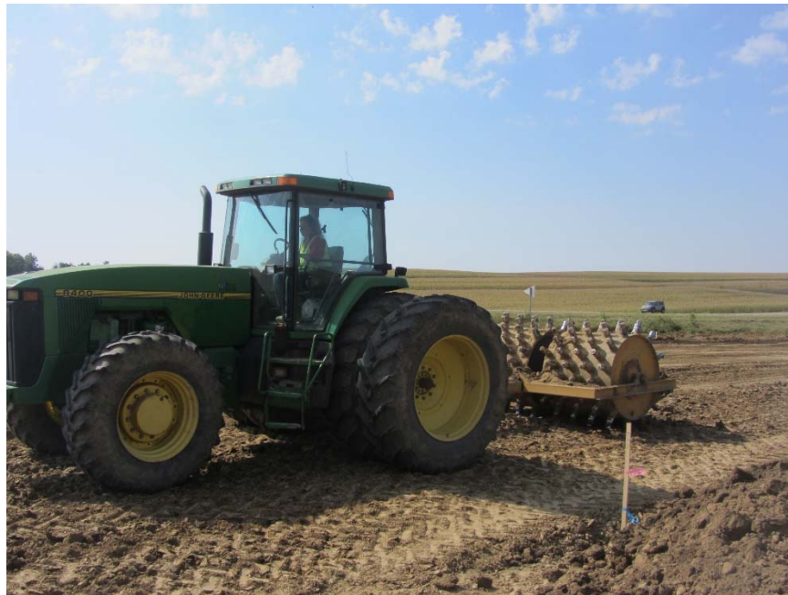
Figure 145. Woodbury County Project 9: Sheepfoot roller used for soil compaction
