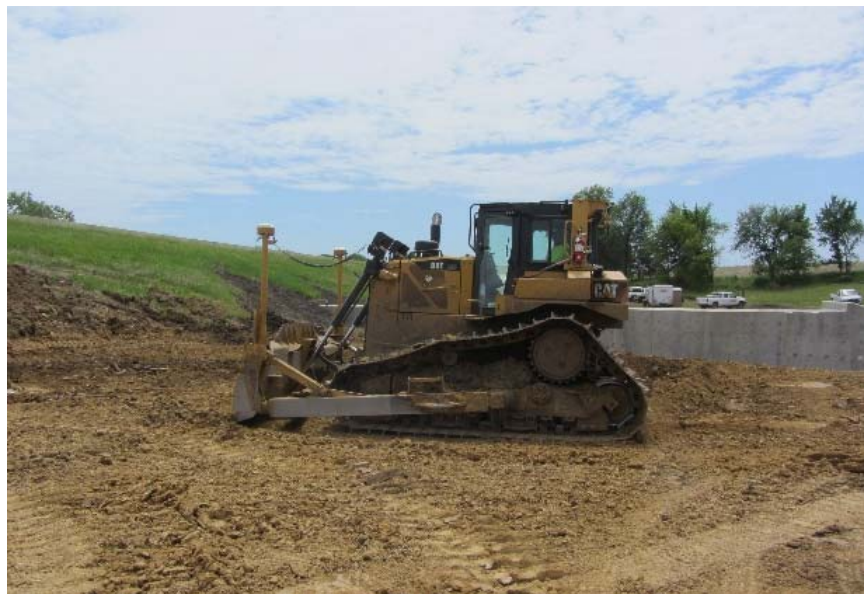
Figure 38. Warren County Project 2: Caterpillar D6T dozer used to control lift thickness
