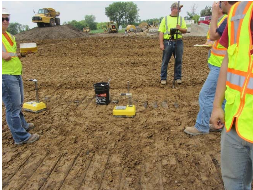
Figure 77. Linn County Project 4: Iowa DOT engineer conducting QA tests
