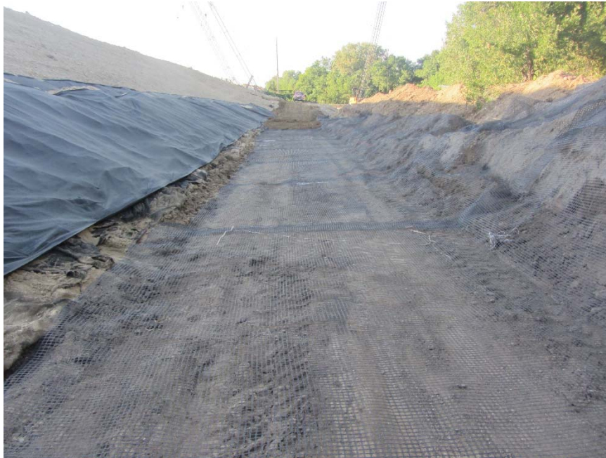
Figure 27. Polk County Project 1: Geogrid placed near embankment toe
