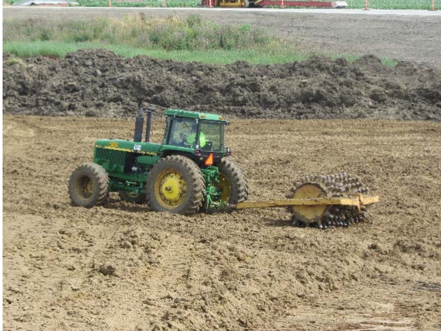
Figure 90. Mills County Project 5: Sheep's foot roller used for soil compaction
