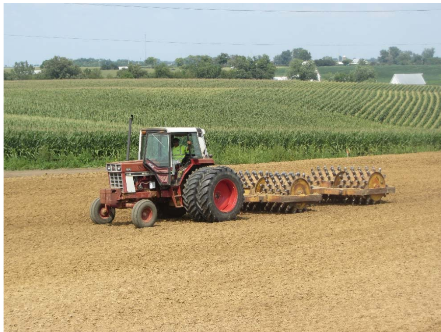
Figure 129. Scott County Project 8: Sheepfoot roller used for soil compaction
