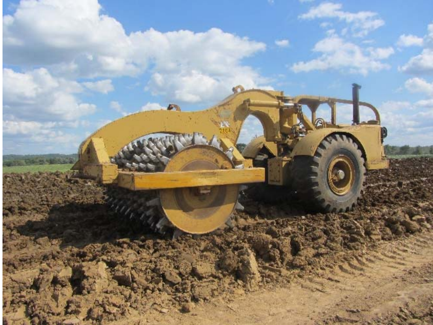
Figure 55. Linn County Project 3: Sheepfoot roller used for soil compaction
