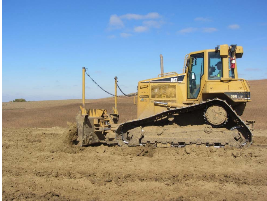
Figure 142. Woodbury County Project 9: Caterpillar D6N dozer used to control lift thickness
