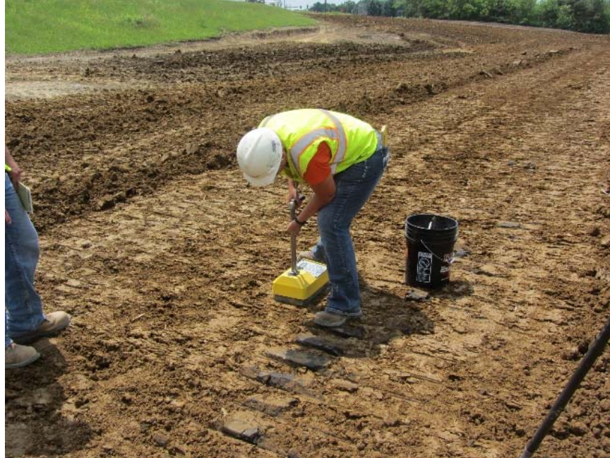
Figure 76. Linn County Project 4: Contractor conducting QC tests
