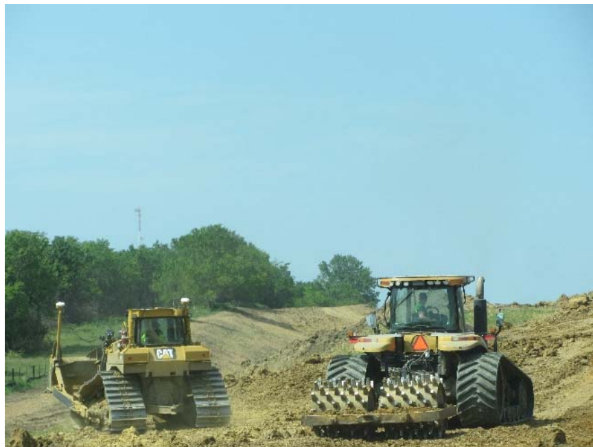
Figure 40. Warren County Project 2: Sheepsfoot roller used for soil compaction
